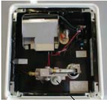
Water Heater Drain Plug
