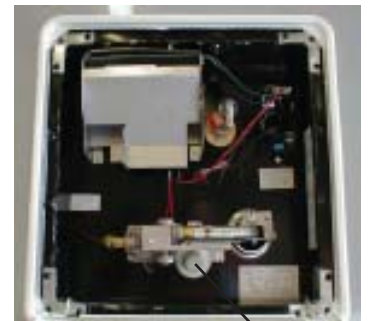
Water Heater Drain Plug
