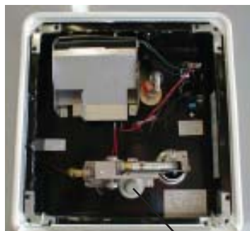
Water Heater Drain Plug
