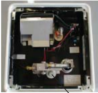
Water Heater Drain Plug
