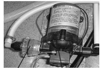
Filter Water Pump
