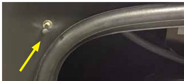
Fuel Pump Safety Lock-out Switch
