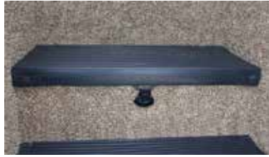
Typical Class C motorhome auxiliary battery location is under the entrance step
