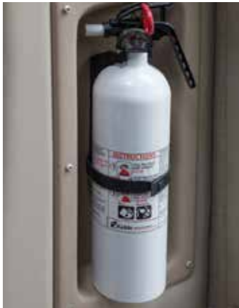
Typical Class B-C fire extinguisher
